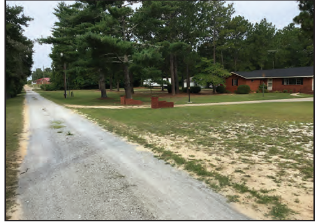
Figure 3.3. Section of Old Plank Road/Old Wire Road Finished with a Layer of Gravel, Located North of Rockfish Road. View Looking Southwest Along Old Plank Road/Old Wire Road Towards Rockfish Road.
